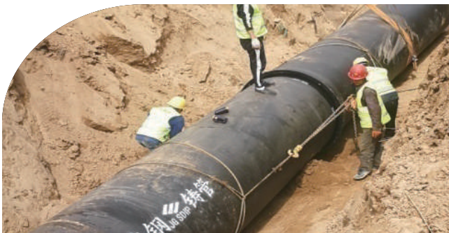
Water supply project of urban and rural West line in Yinchuan metropolitan area Specification: DN 1800 DN2000 34km
