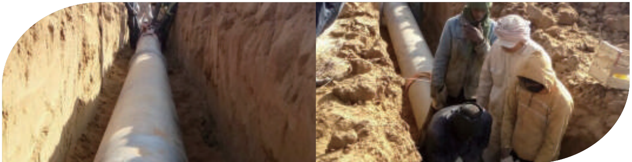
Northern section of the water-supply project Mauritania DN400-DN500: 23,570 TONS
