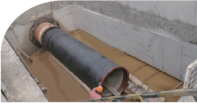
Xixian New Area of Shaanxi Province DN1400 pipe jacking project of sewage reconstruction
