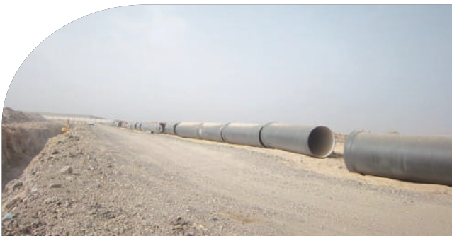
Urban water supply project in Jingdezhen City, Jiangxi Province Raw water transmission pipeline project Specification: DN2000 3km
