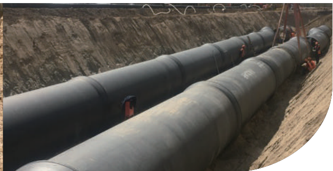
Water supply project of urban and rural West line in Yinchuan metropolitan area Specification: DN 1800 DN2000 34km
